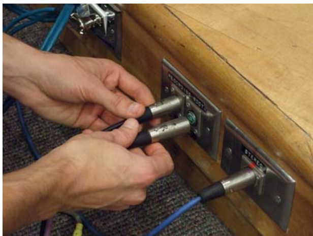
Left and Right are marked. The correct inputs are marked, "recording booth, 1 - 2".
